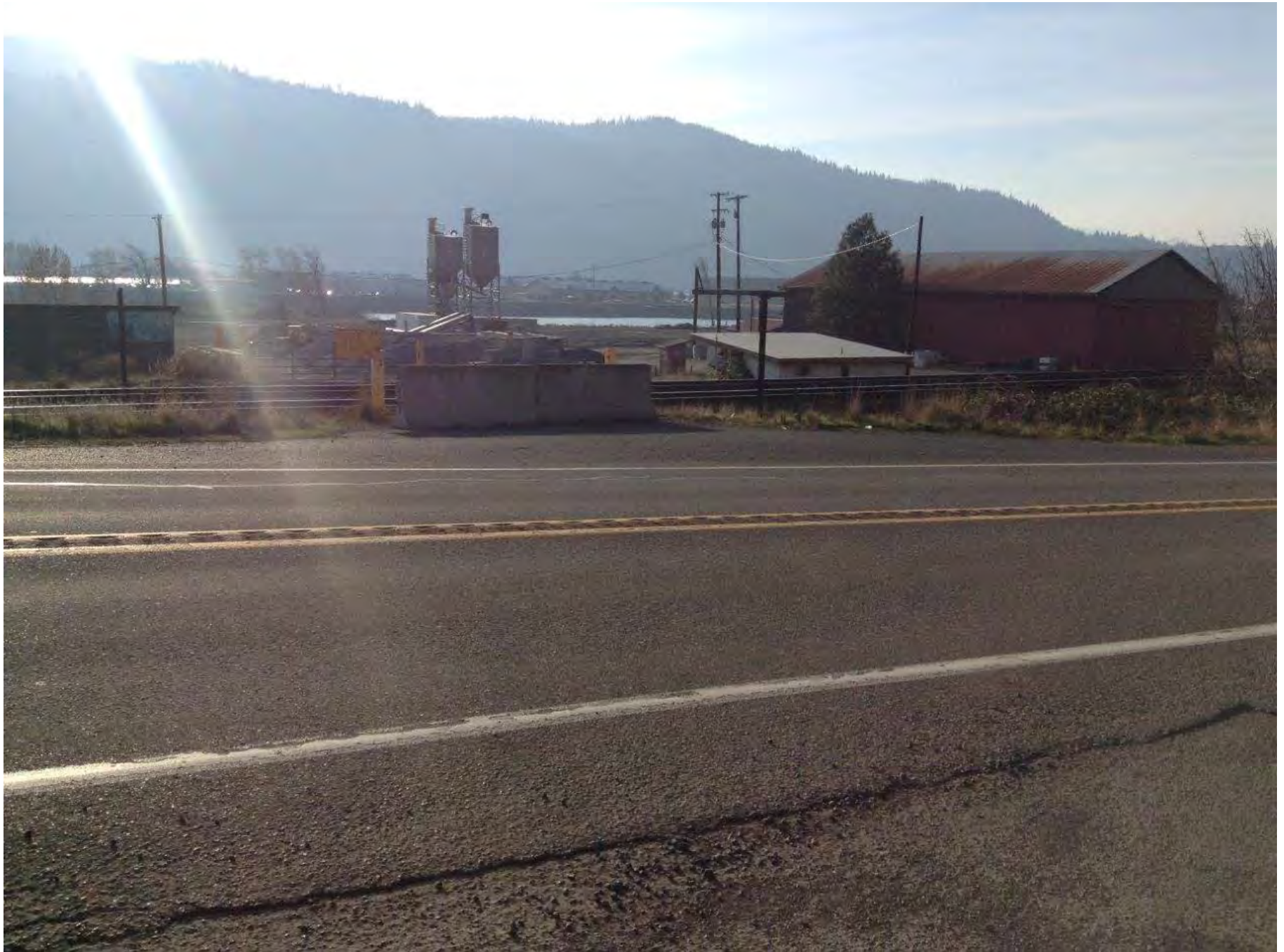
Figures 22. Warner Lane Looking South - Old Crossing
