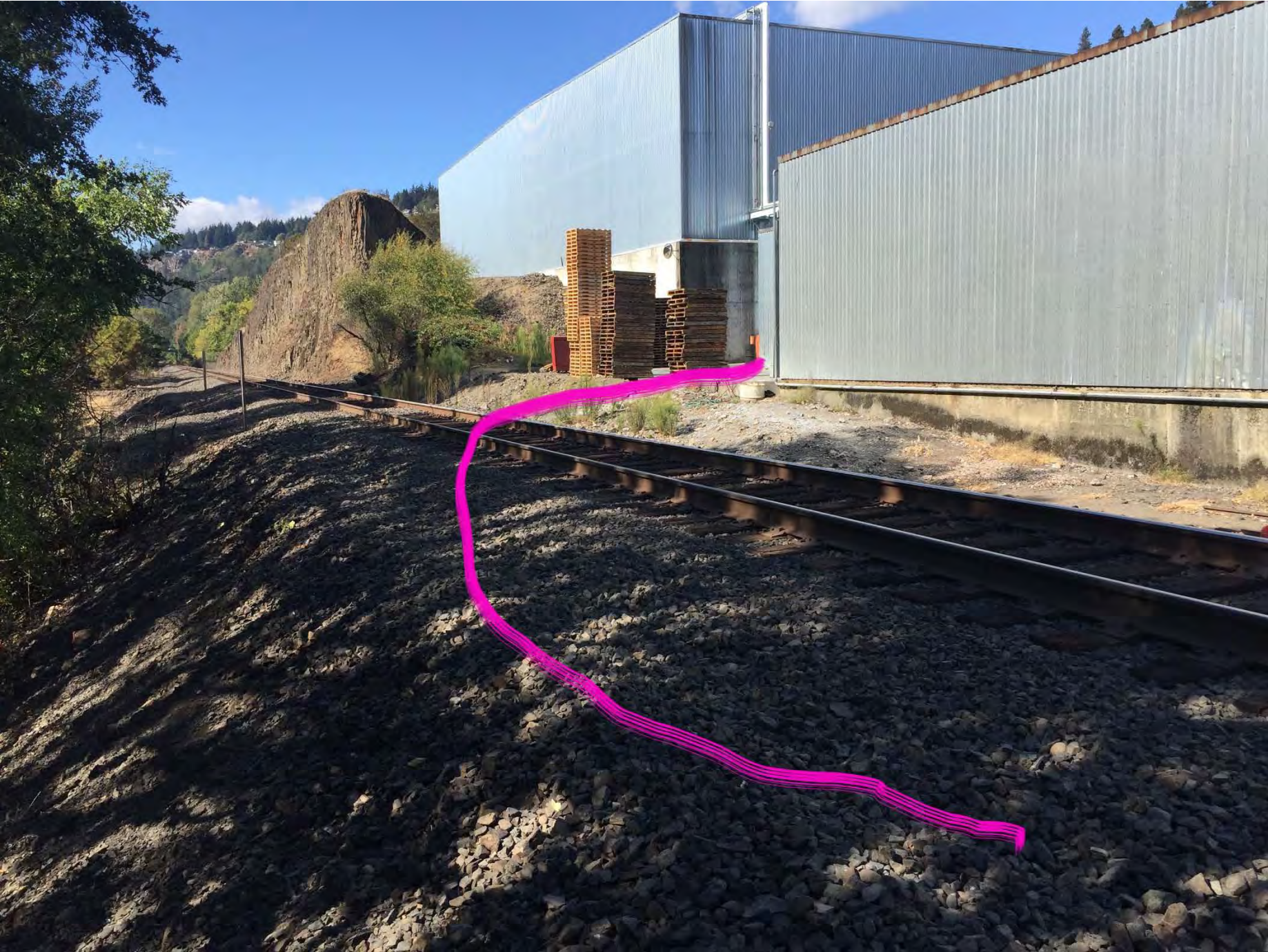
Figures 27. Footpath crossing BNSF Railway from SDS to Mt. Adams Orchard/Underwood Fruit
