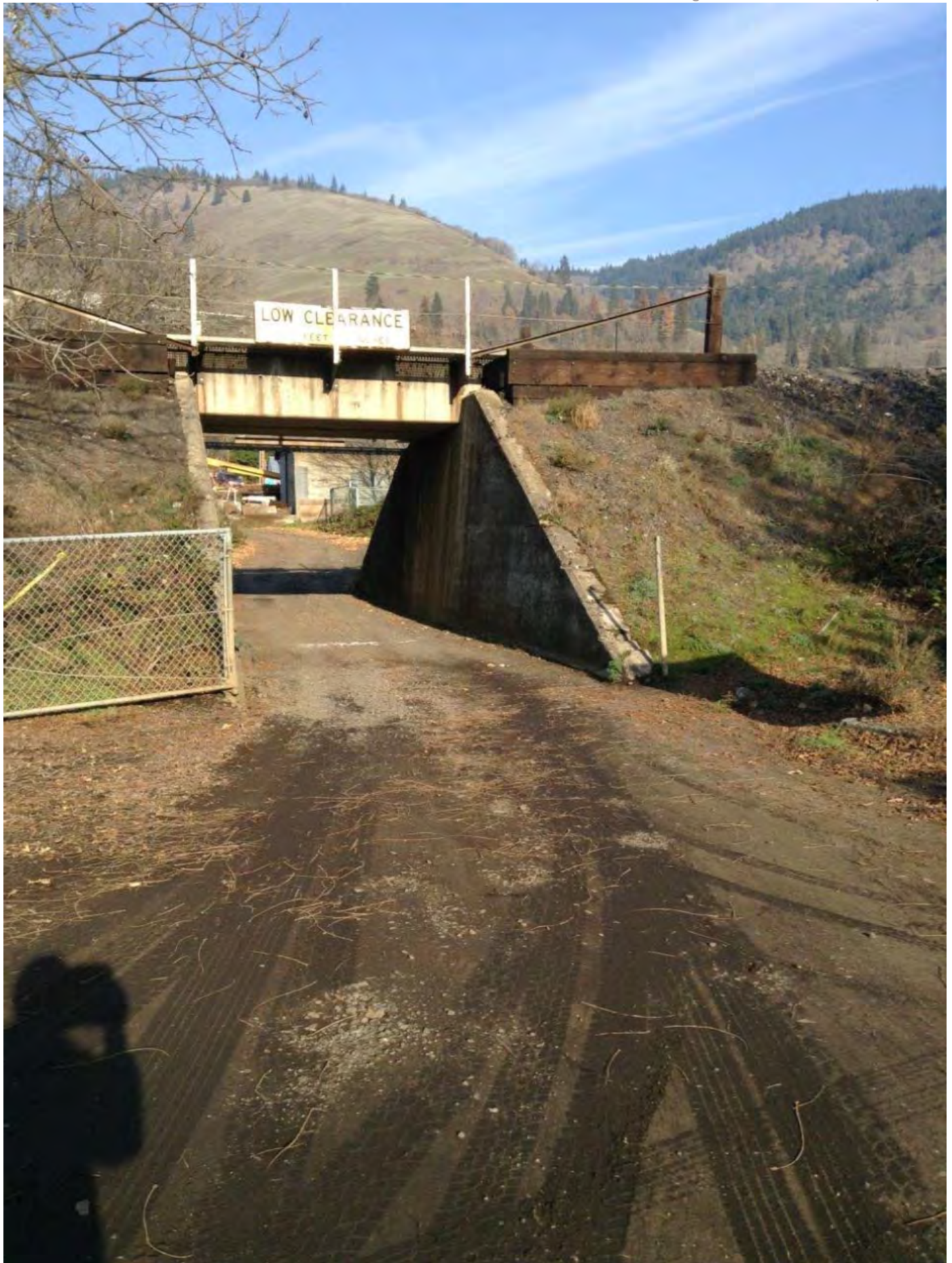
Figures 9. Hearn Drive Underpass Looking North
