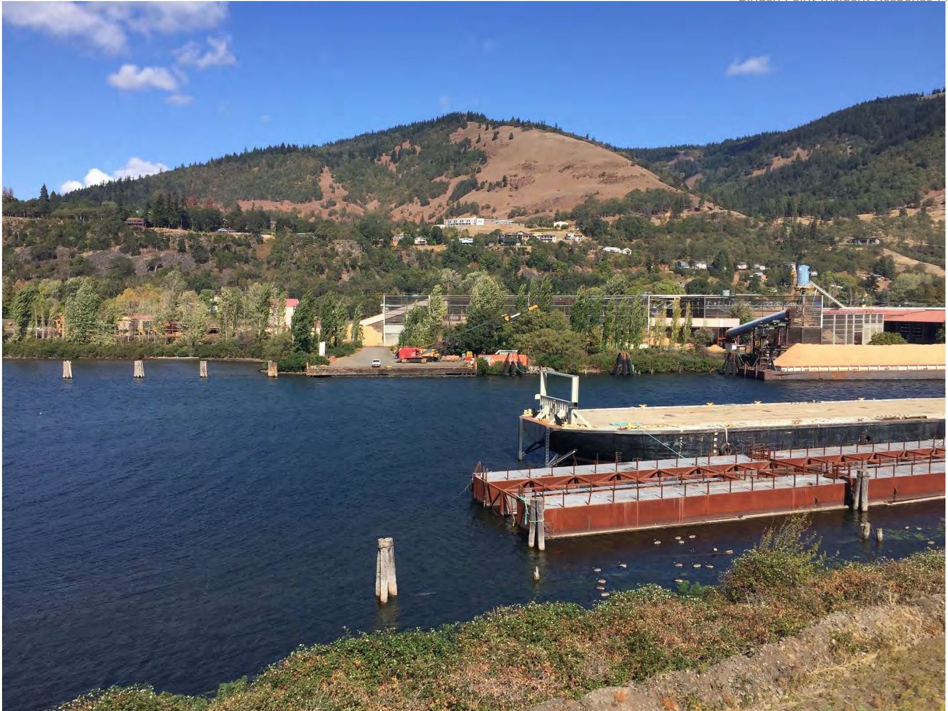
Figures 39. Looking north from south side of SDS Cove at Lower Dock – a recommended small-vessel water evacuation collection point
