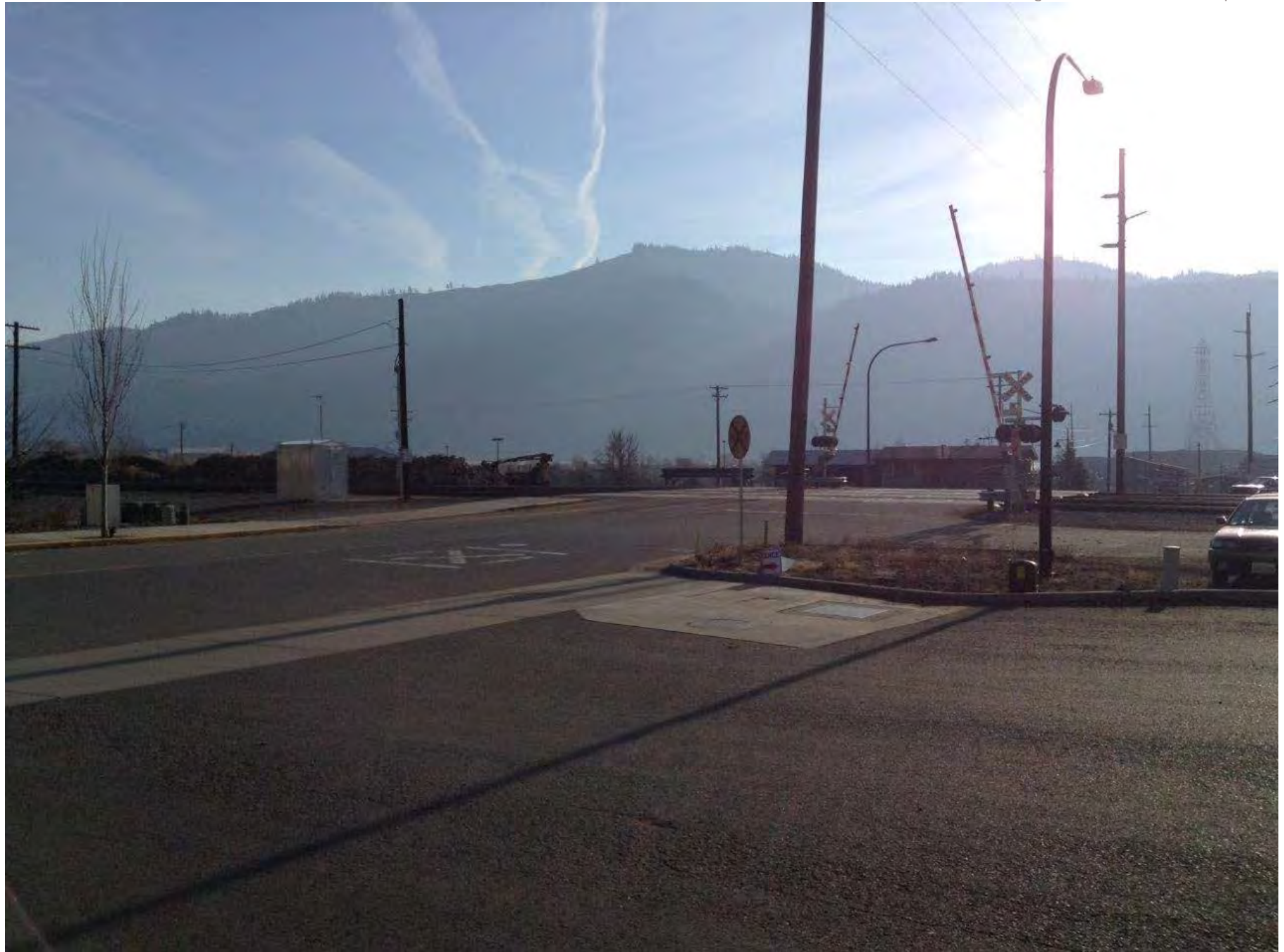
Figures 16. Maple Street Crossing Looking South
