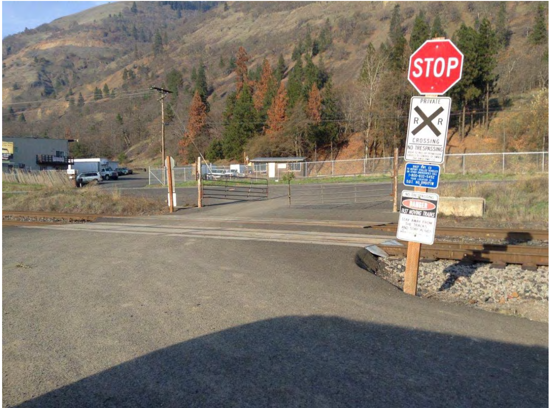
Figures 18. Dickey Farms Road Crossing Looking North
