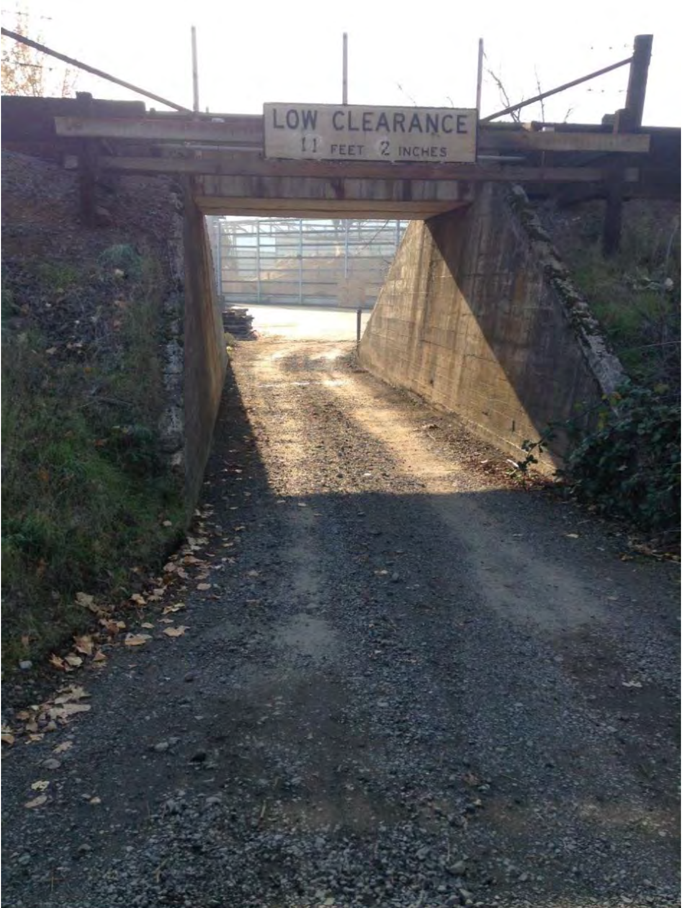
Figures 10. Hearn Drive Underpass Looking South
