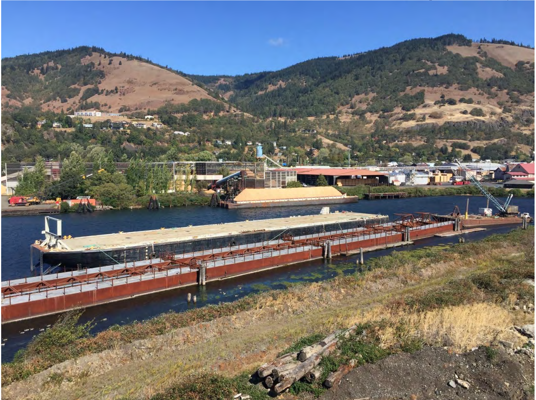
Figures 40. Looking north from south of SDS Cove at Barge Loading Dock – a recommended large-vessel water evacuation collection point
