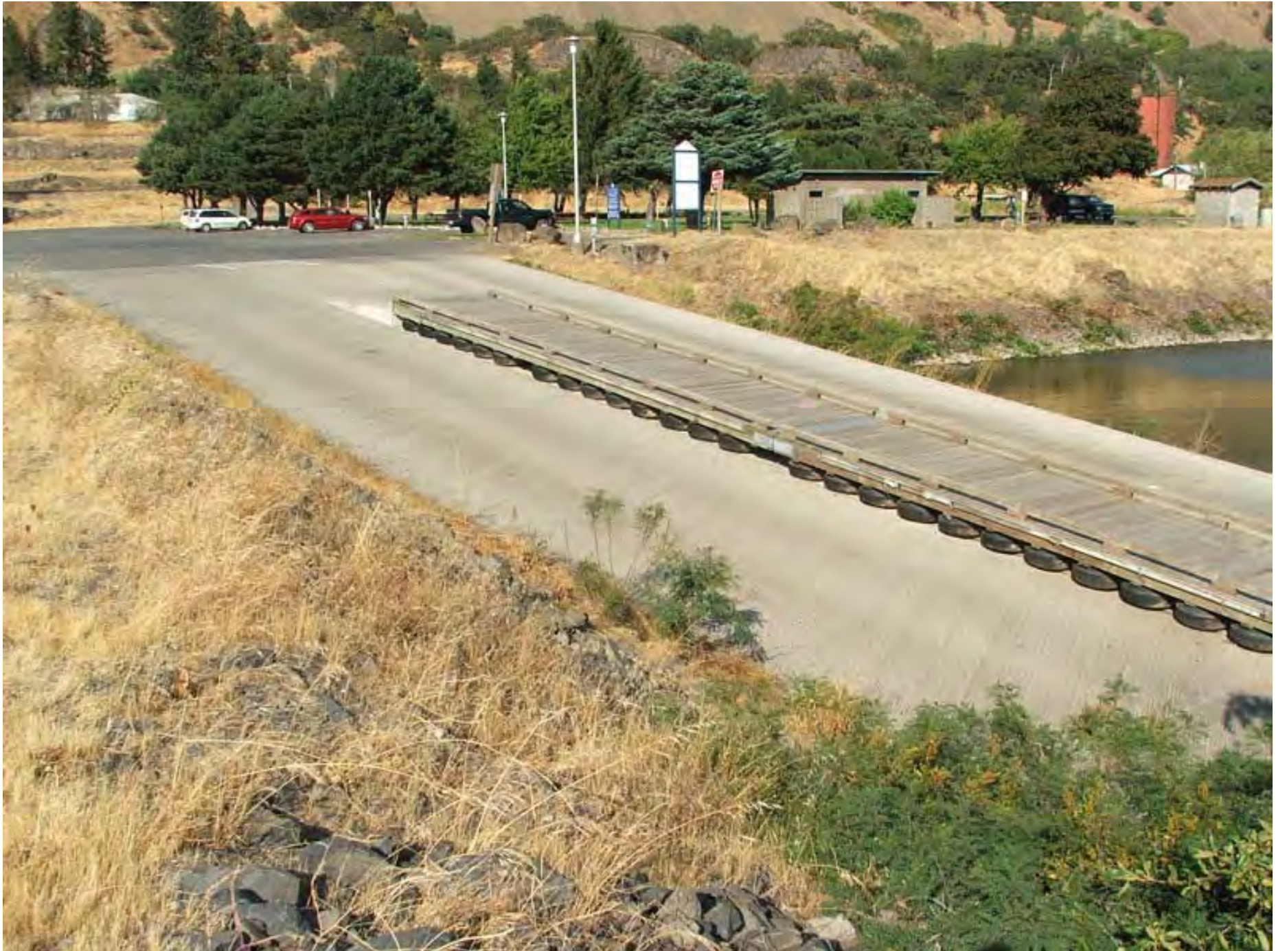
Figures 32. Bingen Marina looking northeast at Marina Park and potential helicopter landing site (parking lot on park's west side)
