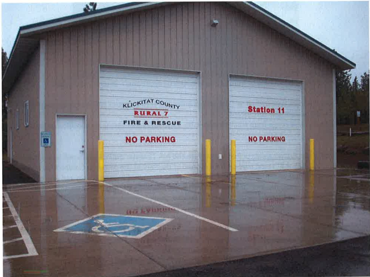
Plate 4.5 Fire District #7 Ponderosa Park Station
