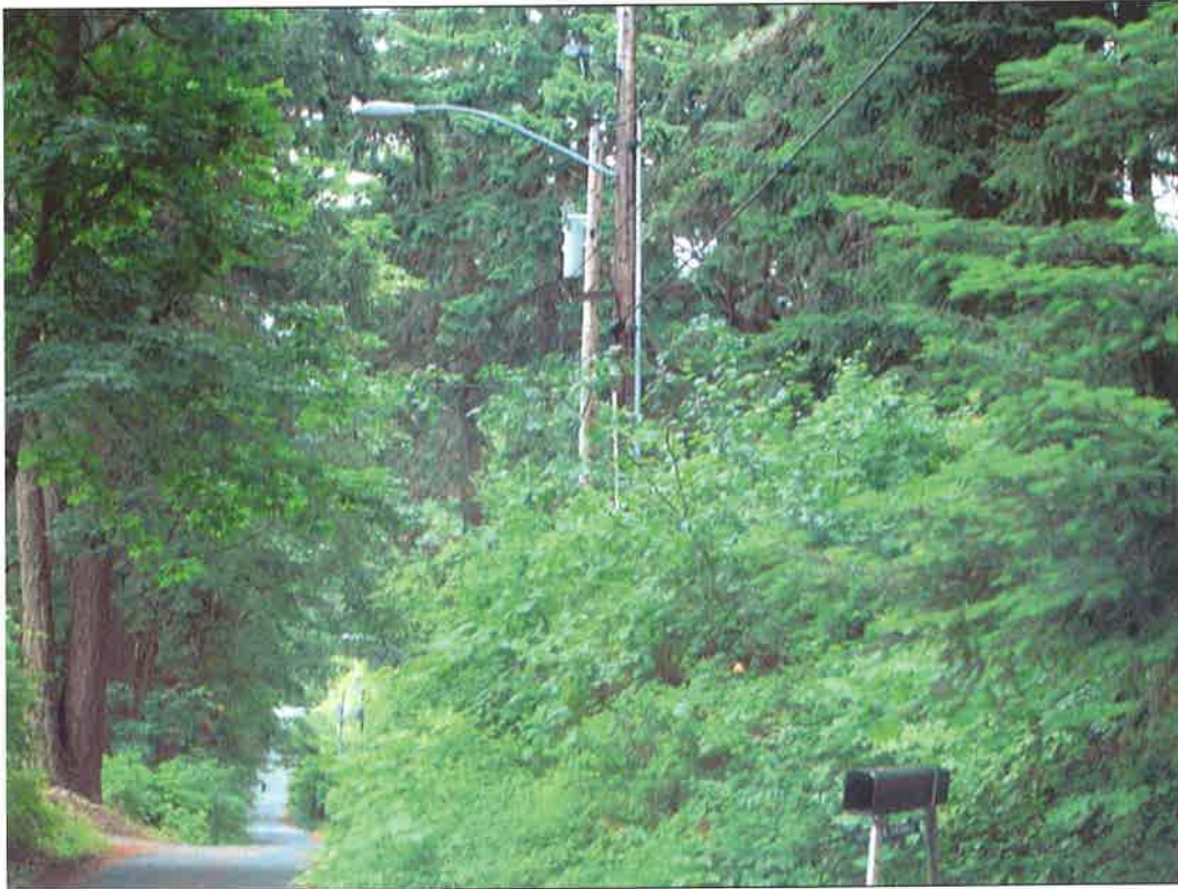
Powerline situated within hazardous fuel situation.
