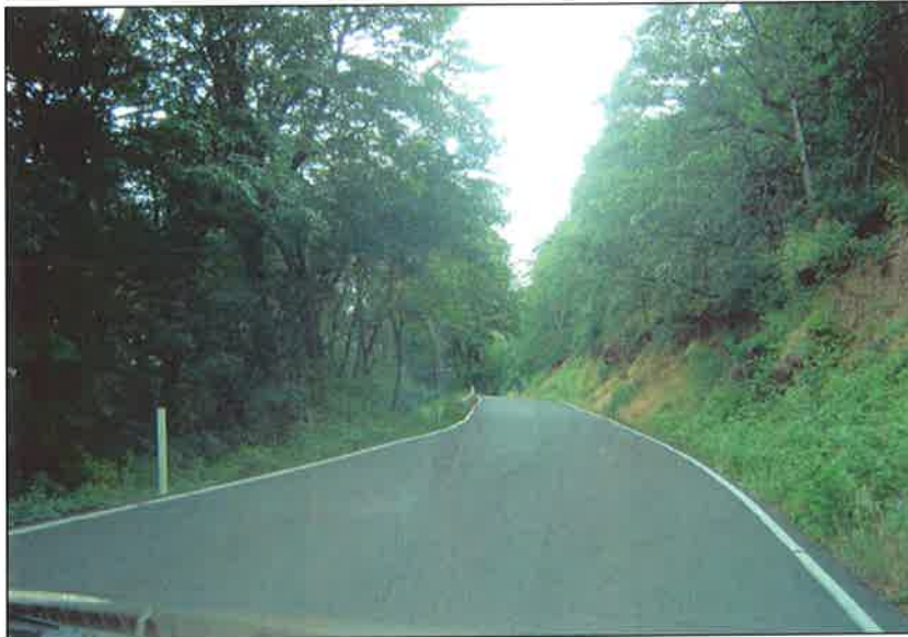
Steep grade and narrow width road (Dock Grade)
