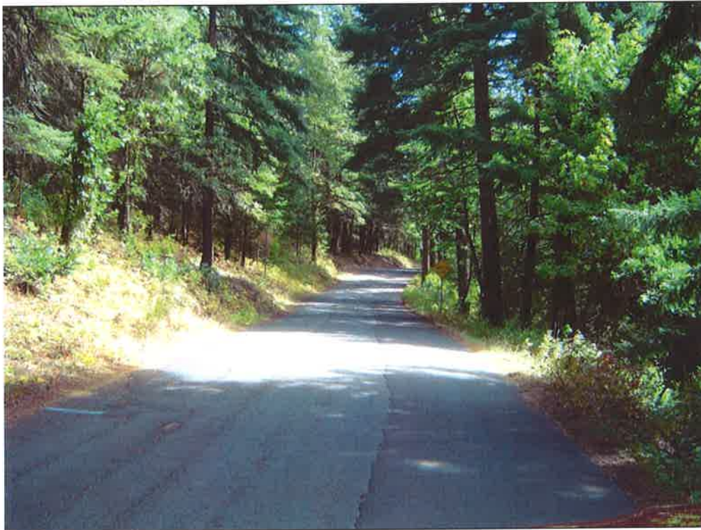
Lincoln Street. Note how vegetation overhangs above the road surface.
