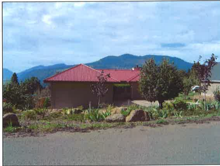
Metal roof, stucco siding. Good example of fire resistant features.
