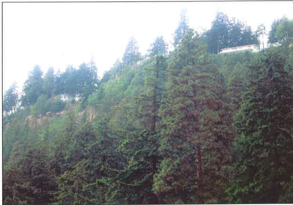
Hazardous fuel and steep slope situation on the bluff above Highway 14. This is an example of a high hazard fuel rating area.
